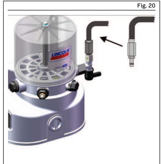
Installing the lubrication piping
